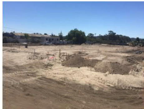
J.W. Design and Construction begins construction on the new 40Prado center!
